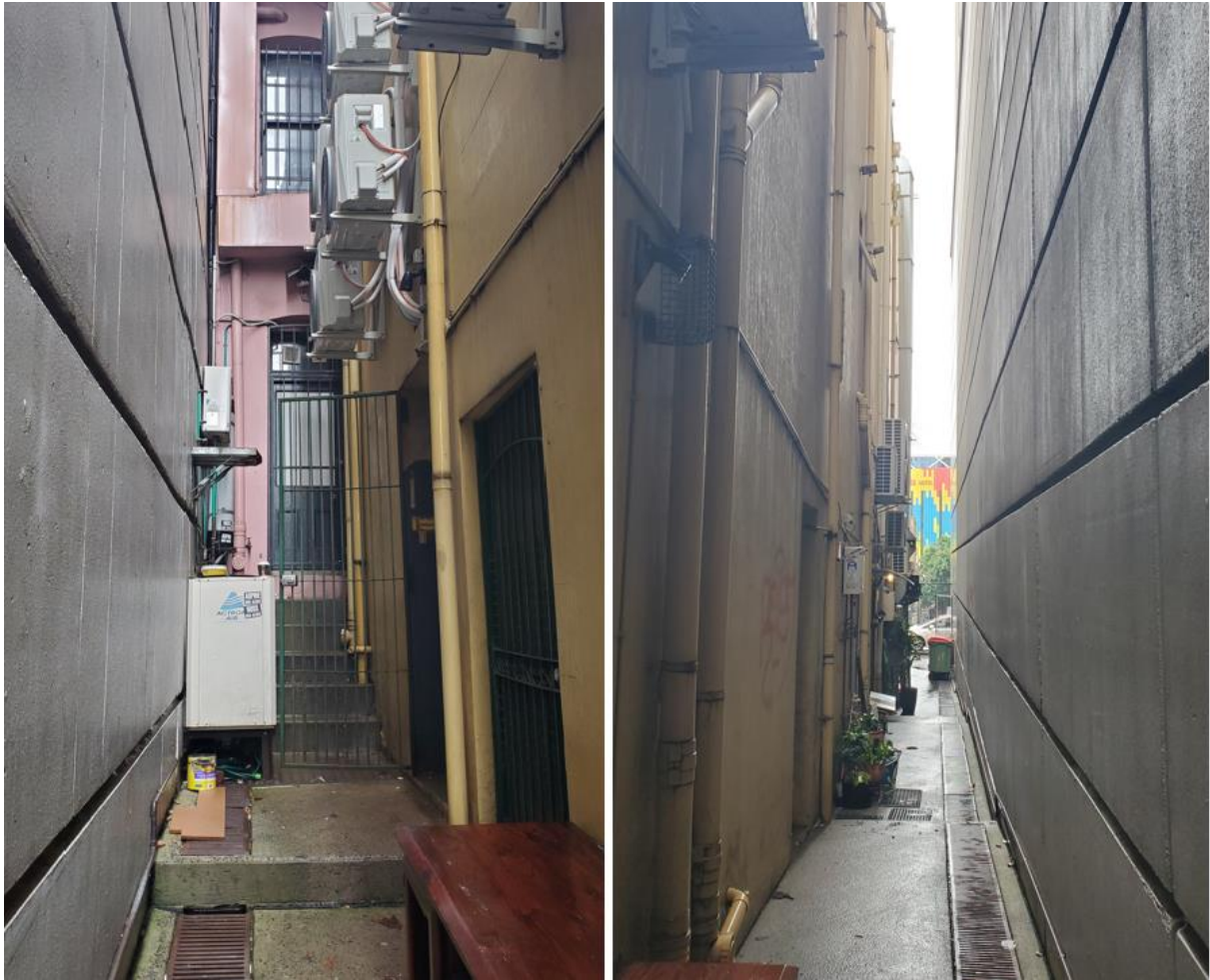
Figure 5: Subject site rear access from Kent Street
