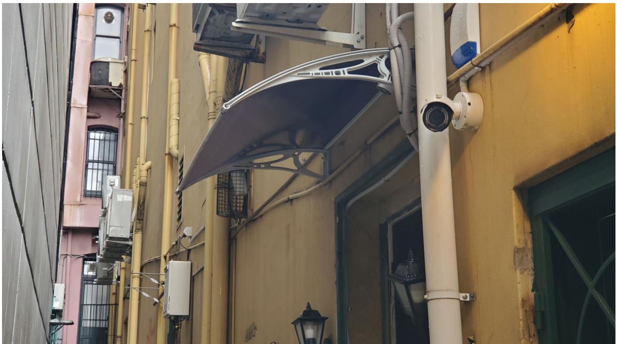
Figure 6: Existing CCTV at 70 Erskine Street with subject site in background
